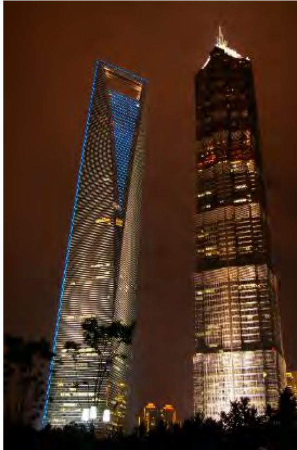
Shanghai Financial Center & Jin Mao Buildings Shanghai, China
