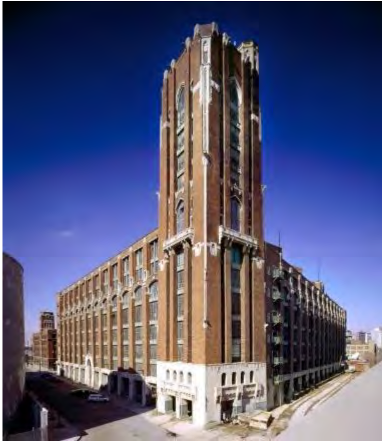
Lakeside Technology Center Chicago, IL
